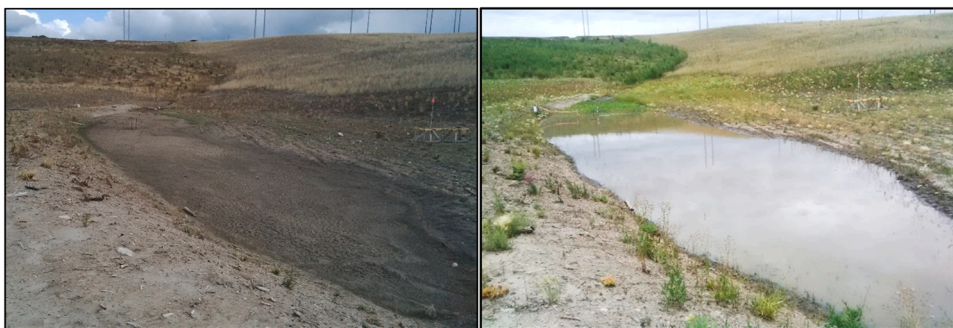
Fig. 2. East recharge basin empty (left) and full shortly after a large rain event (right). Photos taken in May 2015.
