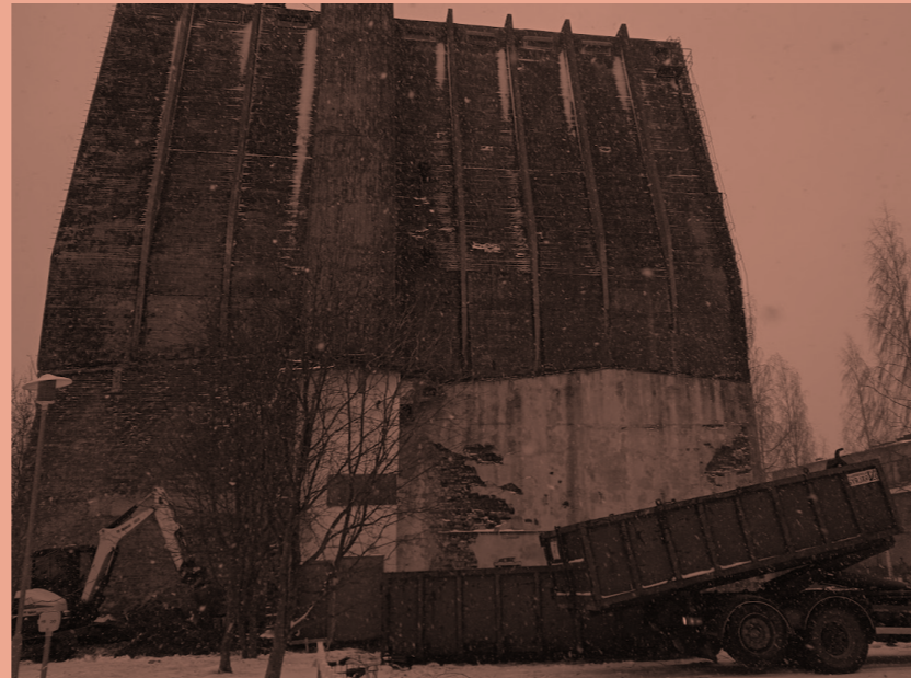
△ Fig 51. Cleaning of the plot
