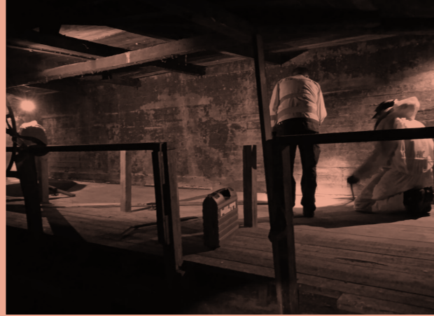
△ Fig 52. Fixing of the original hoppers bridge
