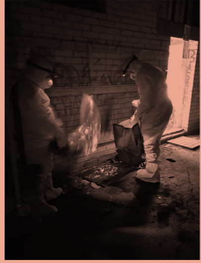
△ Fig 50. Workers taking out metal pieces from the interior
