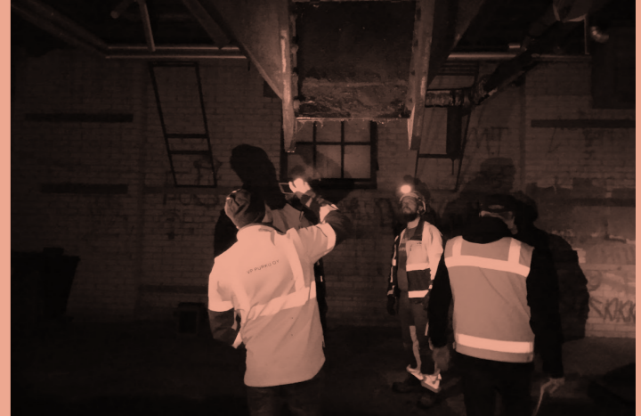
△ Fig 56. Demolition team specialist visit
