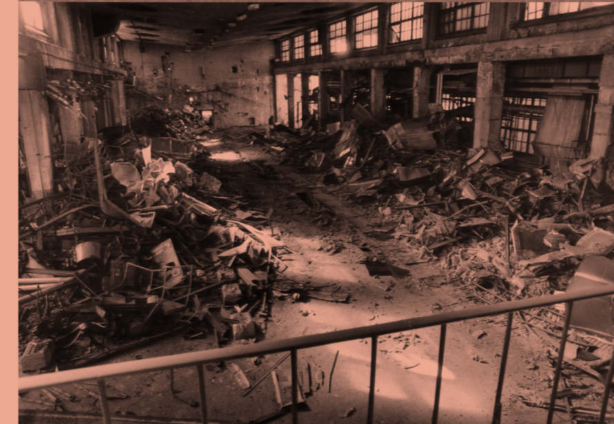
Fig 19. 1993 demolished part adjacent of the Silo
