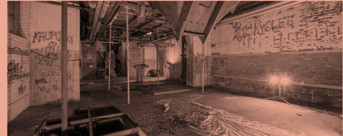
Fig 29. Groundfloor of the Silo ▷
