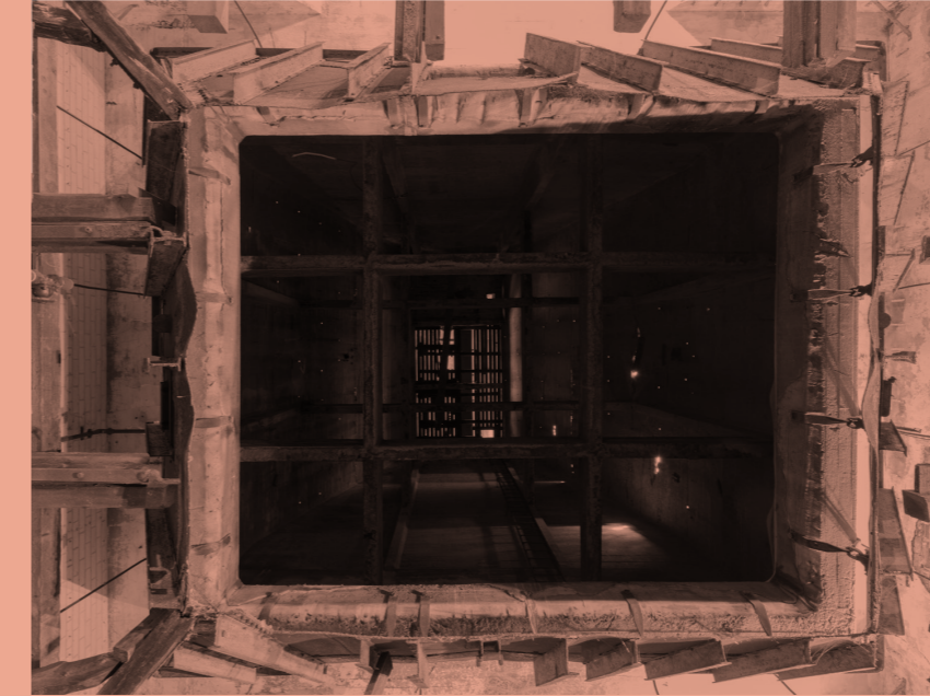
△ Fig 27. view from below one of the Silo hoppers
