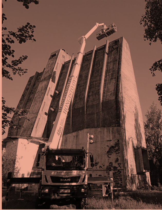
△ Fig 46. Roof inspection and minor works
