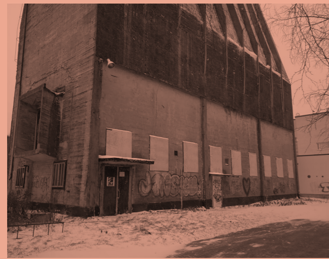
△ Fig 47. Provisional panel protection for broken windows and doors
