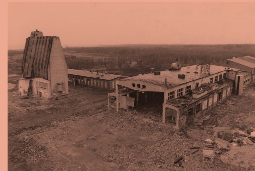
Fig 20. 1993 demolishing jobs on the Silo
