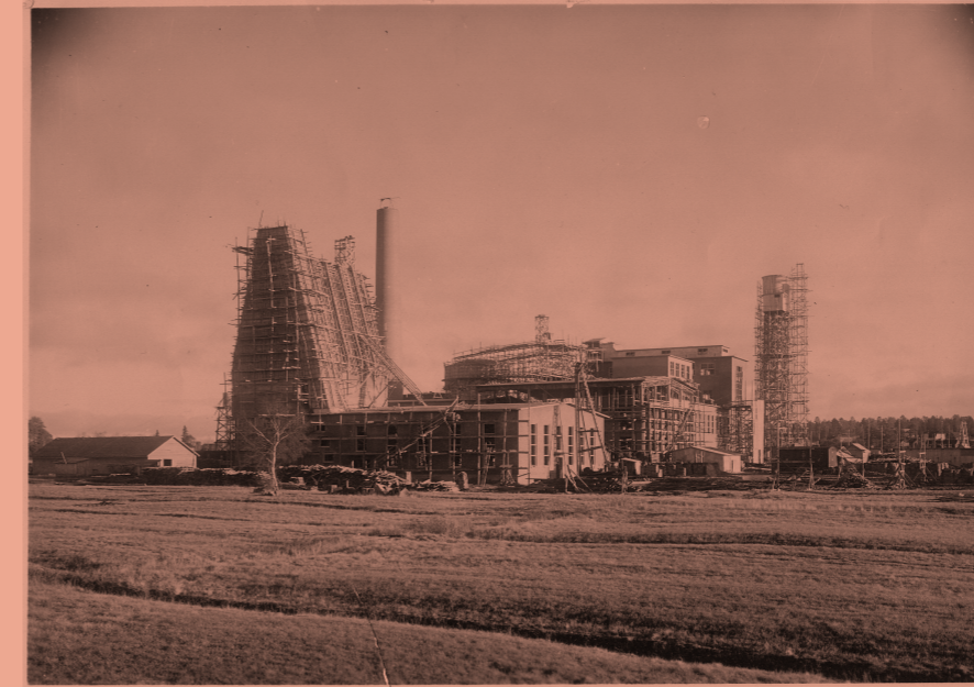
Fig 16. Silo under construction in 1931
