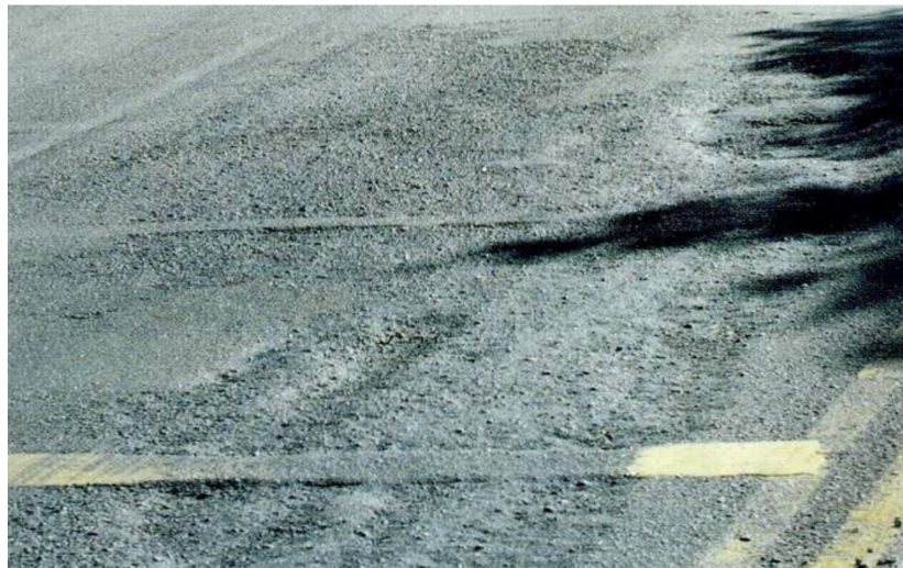
Figure 6.4: Material movements in the pavement example - ravelling (adapted from Research & Development division of the Highway Department (2013) ).
