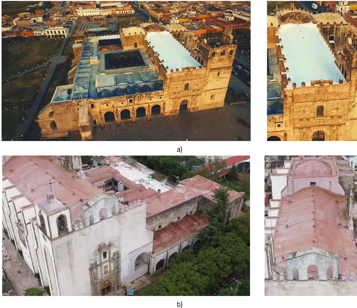
Figure 2-18. Extrados as a flat surface interrupted only by the longitudinal elevation of the crown of the vault: a) Yuriria, Guanajuato (Wallfisch, 2016); b) Atotonilco el Grande , Hidalgo (Hernandez, 2019).
