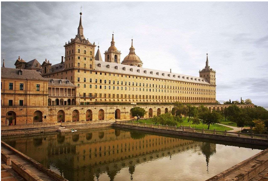
Figure 2-5. Examples of Purist style architecture in Spain: monastery of San Lorenzo at El Escorial (Segundo, 2009).
