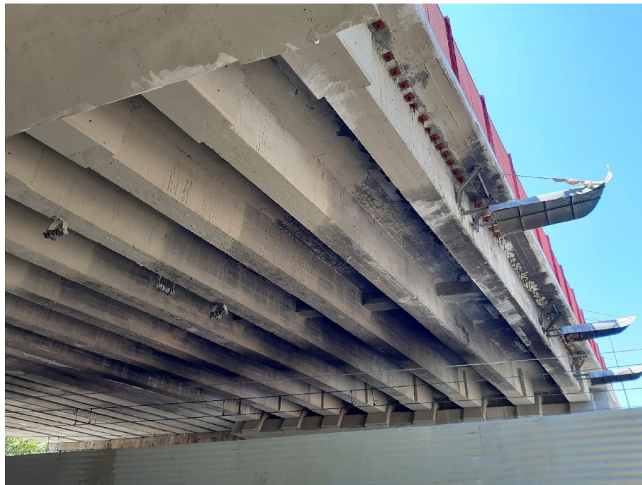
Figure 8. Road bridge analyzed.
