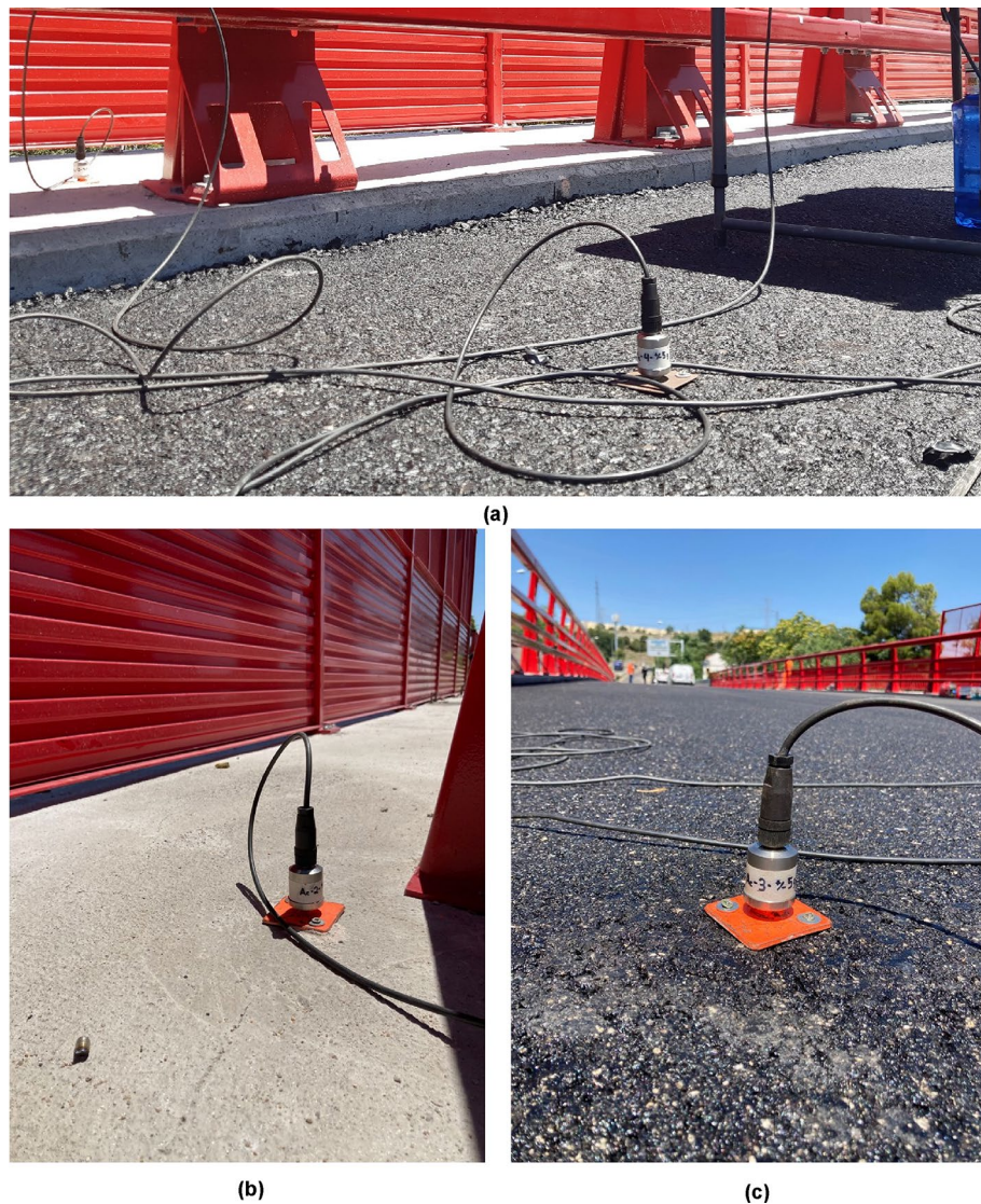
Figure 11. Piezoelectric accelerometers used in road bridge dynamic load test: (a) piezoelectric accelerometers on girders 1 and 2; (b) piezoelectric accelerometer on girder 8; (c) piezoelectric accelerometer on girder 7.
