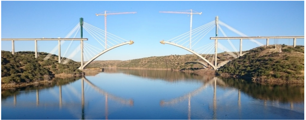
Figure 1. Tajo River Viaduct during its construction.
