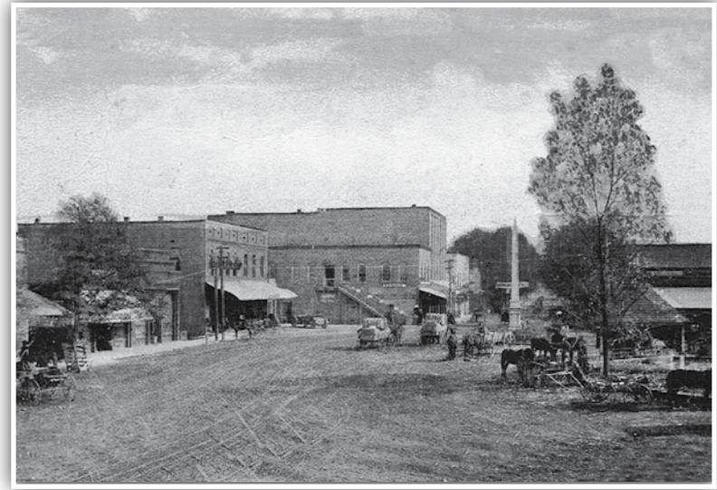
Public Square, circa 1919. Note the electrical power lines which have now been installed.
