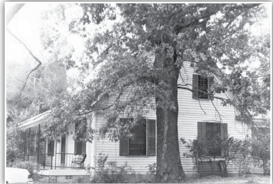
Paris Simkins house No longer standing - demolished 2000
