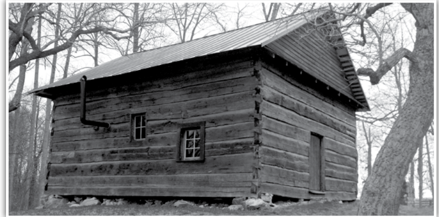
Sandy Creek Church building constructed in 1802
