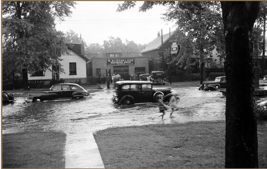
Horton Street Flooding, 1950, 8322, Ron Nelson Photography Ltd Collection, ASCWU.
