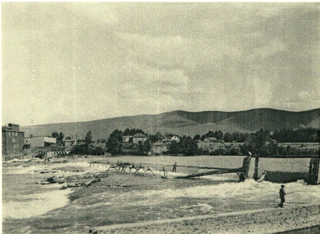
Figure 9. Prosser Dam--1923. Notice the absence of fish ladders. (Source--NADC)
