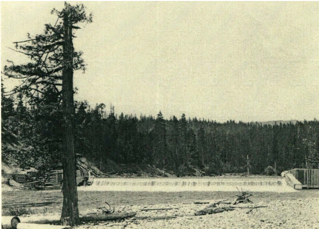
Figure 6. Crib dam at the outlet of Lake Cle Elum, 1923. Box-like structure on the right side of the spillway may be a fish ladder. (Source--NADC)
