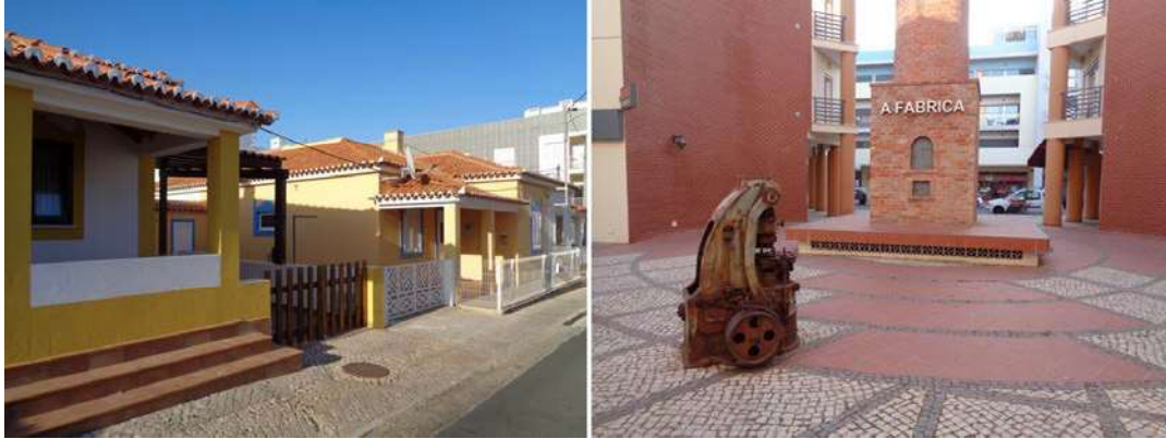
Figure 5: Left: Working quarter; right: some of the remaining elements of the old Mercantile factory (authors)
