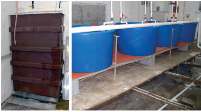
Figure 2. Existing equipment may be retrofitted for aquaculture production: (a) Flush tanks can be converted to biofilters, and (b) racks can be used to support fish-rearing tanks.
