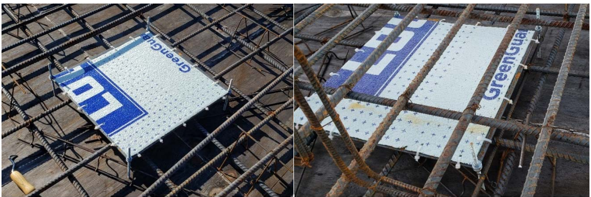
Figure 4-4: Details of mounting defects with 4-in deep in the concrete slab: A steel frame was used to mount delamination at the middle of the concrete slab.
