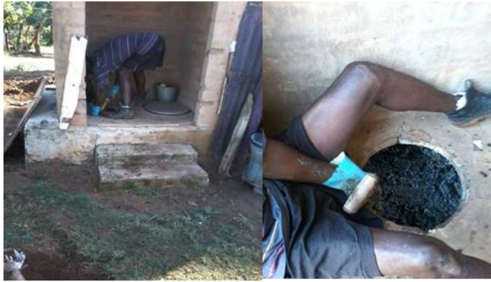
Figure 4.3: A man removing the sludge from the vault inside the UDDT without proper PPE
