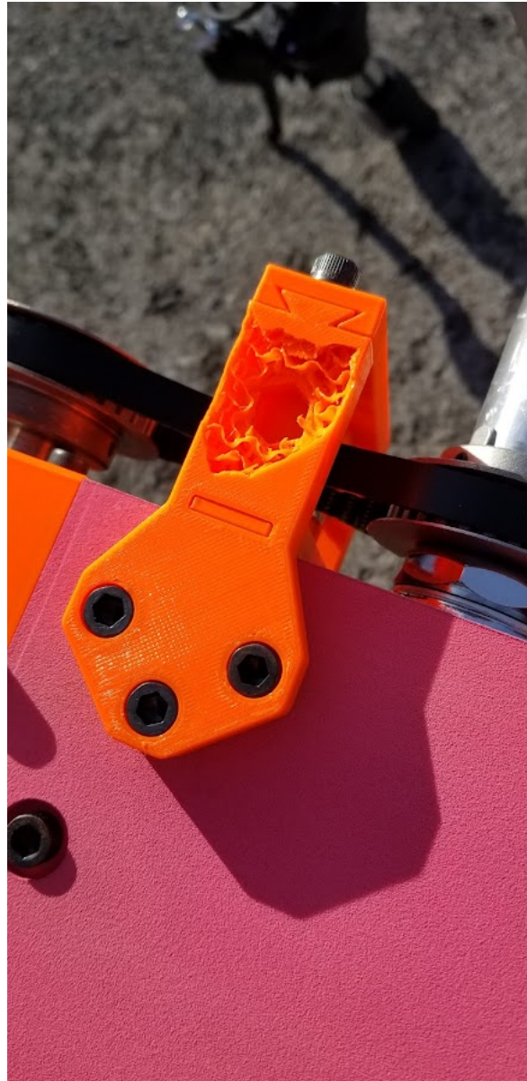
Figure 4.8: Bolt tearout as a result of the Autocycle falling over during initial field tests. This test demonstrated a need for a tensioner robust to impact loading.
