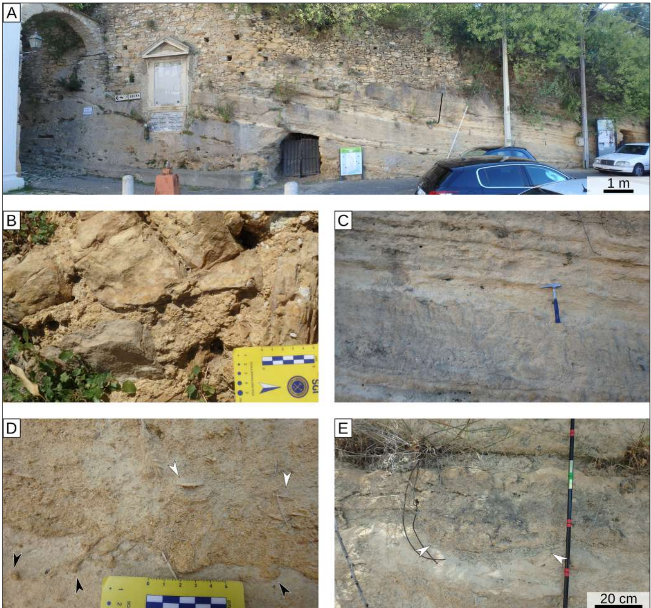
Fig. 6 - Section S3. A) Overview of S3 from the church square. B) Detail of the basal breccia layer of S3. C) Overview of the fine-grained calcirudite layers from the upper part of S3 alternating with calcarenites. D) Detail of a fine-grained calcirudite layer displaying a thoroughly bioturbated base (black arrowhead); white arrowhead = bivalve shells. E) Fine-grained calcirudite layer filling a scour carved into the underlying calcarenites; white arrowhead = cut-and-fill structure.
