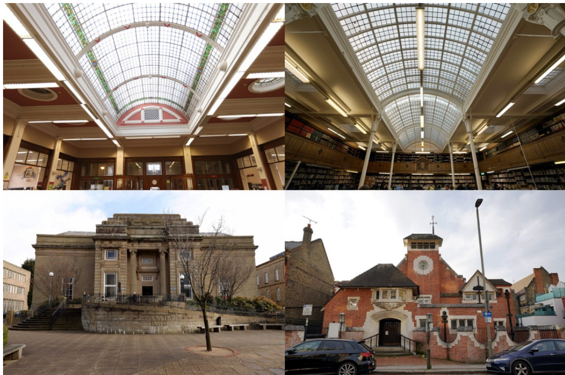
Figure 1. Left: Burnley Library Facade and Interior, A Race, 1930 Right: Battersea Reference Library Façade and interior, H. Hyams, 1924.
