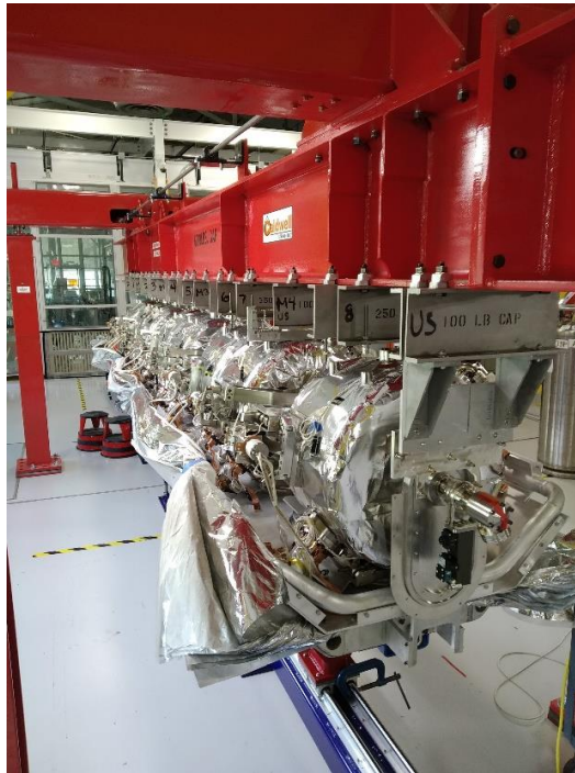
Figure 2. Cavities, thermal shield and strongback accessible for sensor placement.
