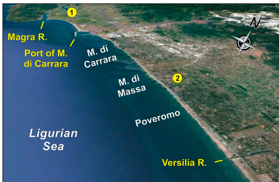
Figure 5. Aerial view (GoogleEarth database) of the northernmost sector of the study area (sub-cells 1 and 2), from the Versilia River mouth to the Magra River mouth. The image is tilted, so the scale is not uniform: as a reference, the distance between the Magra River mouth and the Versilia River mouth is about 14.5 km.
