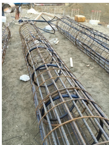
Fig. 2. The installed heat exchanger in EP2.
