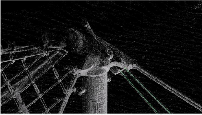
Figure 4 Point cloud from the roof cable net. Detail of mast and cables. Source: sbp
