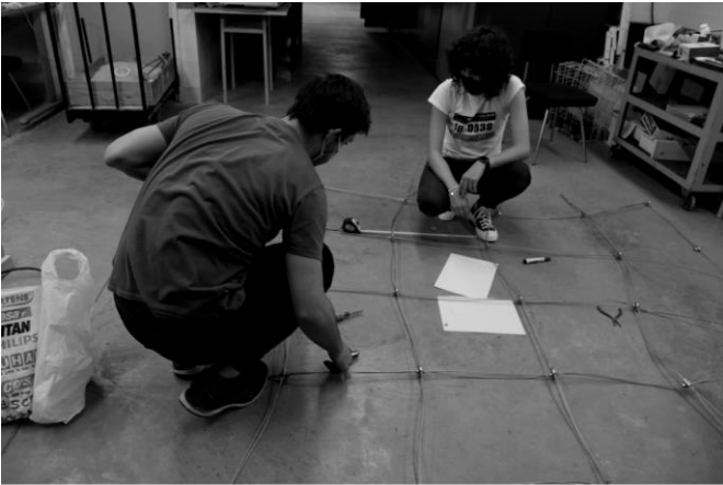
Figure 6 Organization of the cables before tensioning. Source: Authors
