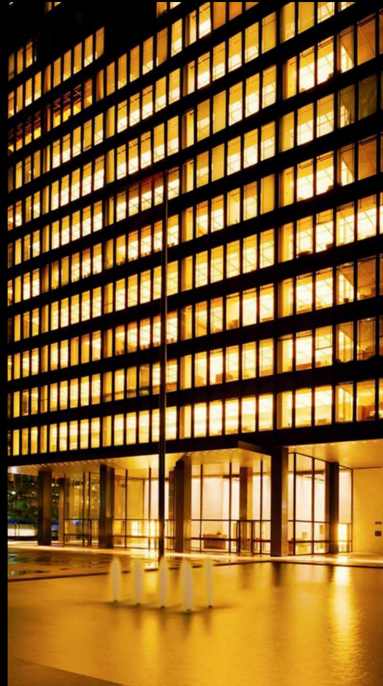
Fig: 303C | View outside the building
