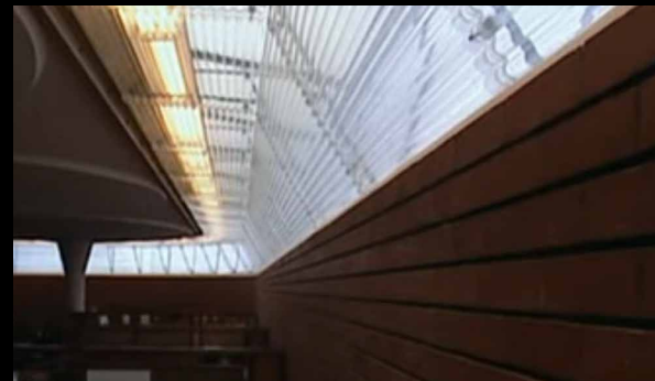
Fig: 305B | View of the lateral openings
