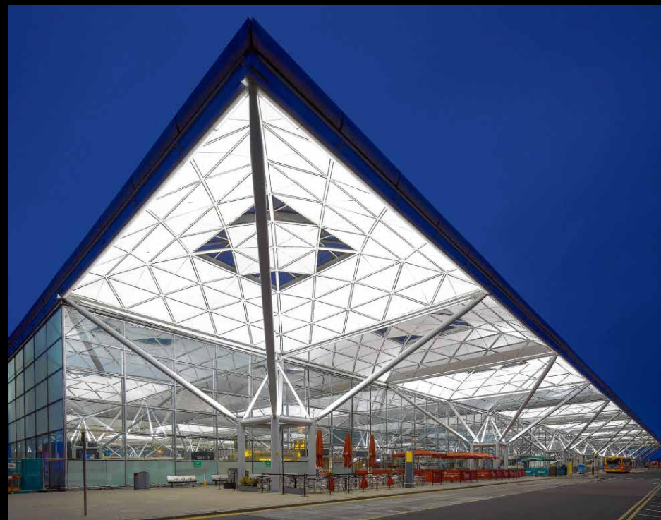
Fig: 304A | View of the illuminated entrance porch
