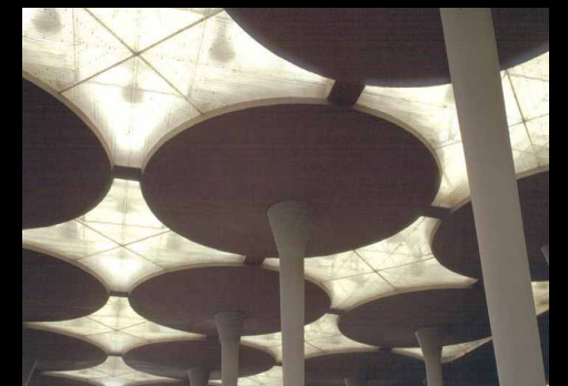
Fig: 305E | View of the light sources that are integrated in the building's zenithal solar windows
