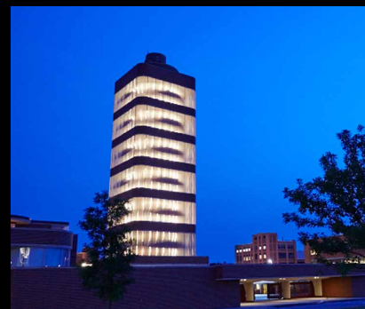
Fig: 305D | Outside view of the building
