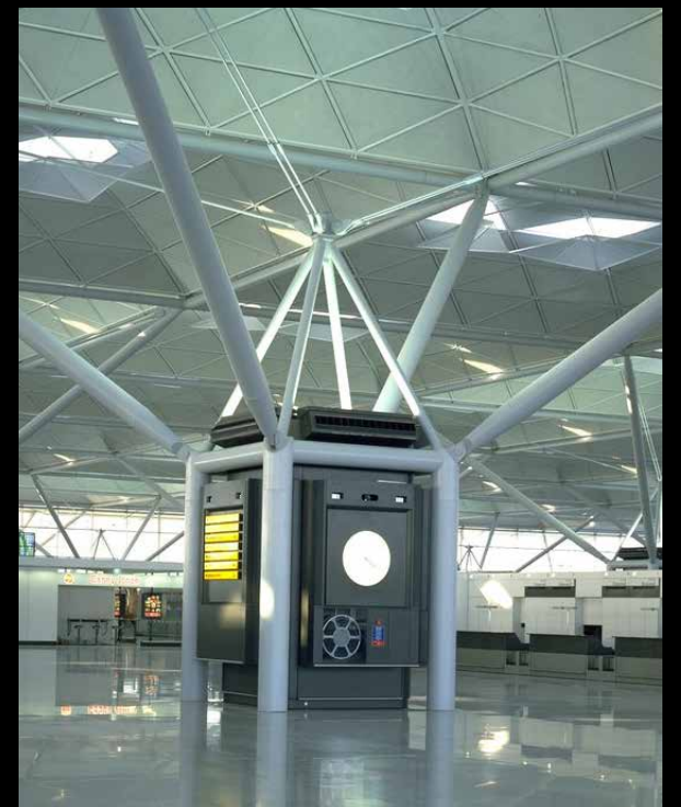
Fig: 304C | interior view of the estructure of terminal
