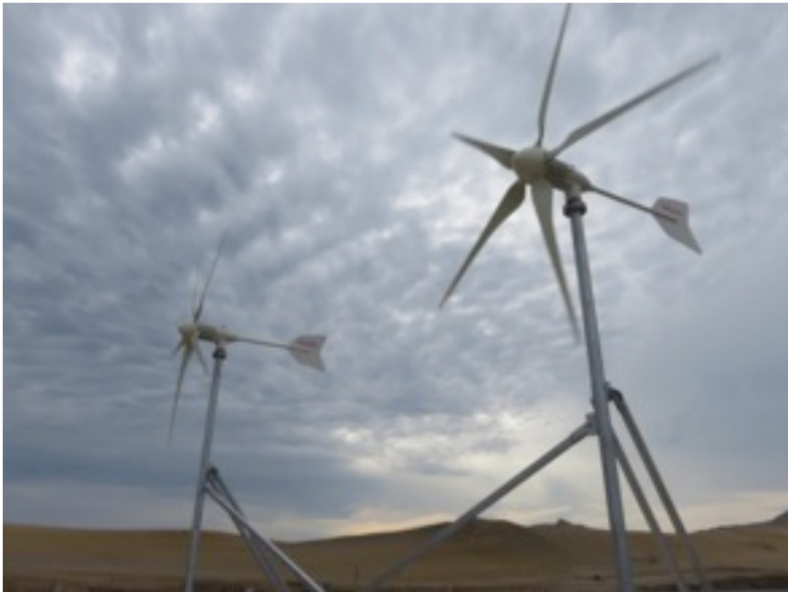
Figure 26: Two 3 kW wind turbines with 3m diameter rotor with 5 blades on the roof of the Laguna Grande community building
