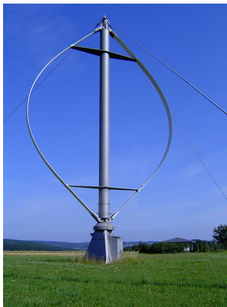
Figure 1.3.2: Layout of a VAWT
