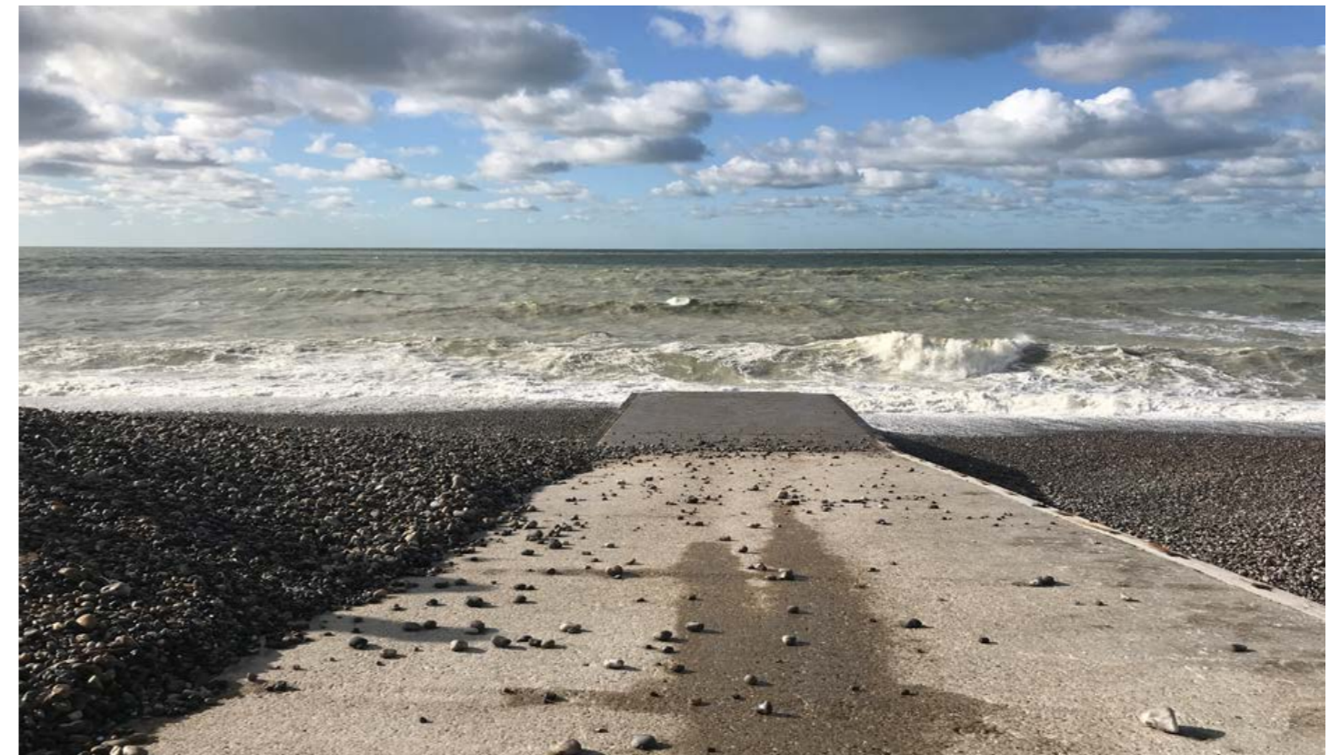
Photo by L. Samson : we can see the accumulation of the pebbles on the south side and the erosion on the north side. this is because the migration of sediment happens from south-west to north-east
