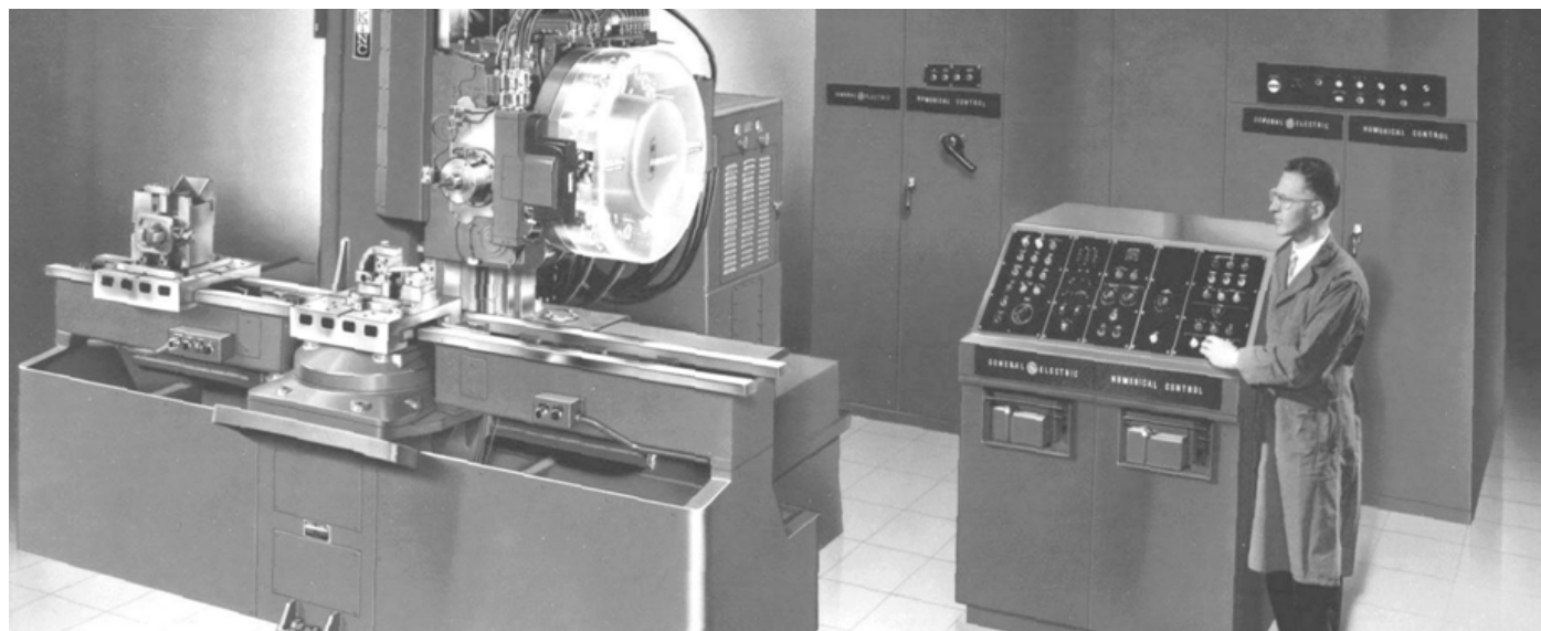
Fig. 4.2 First Control Numerical Machine developed by Parsons [18].
