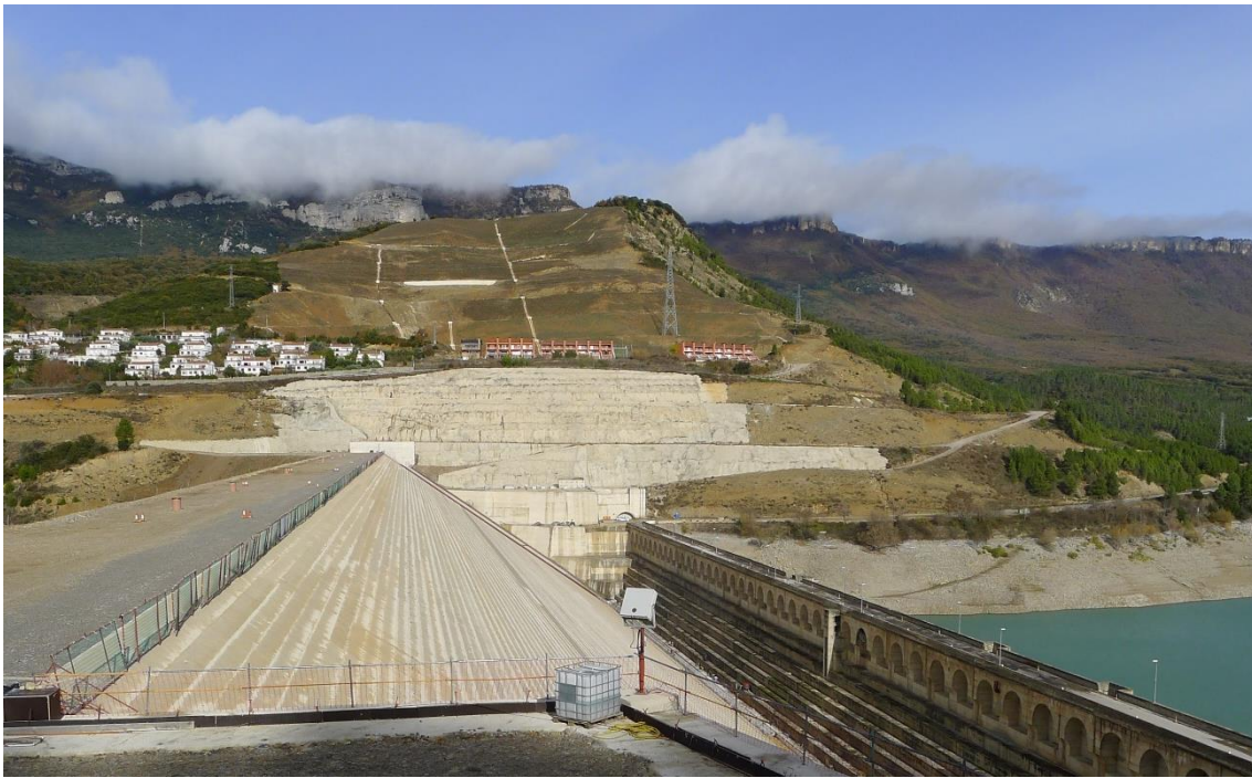
Figure 5.1. The old and new Yesa dams and the landslide in the background.
