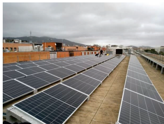
Fig.5. Installation of PV system at the roofs of buildings A classrooms.
