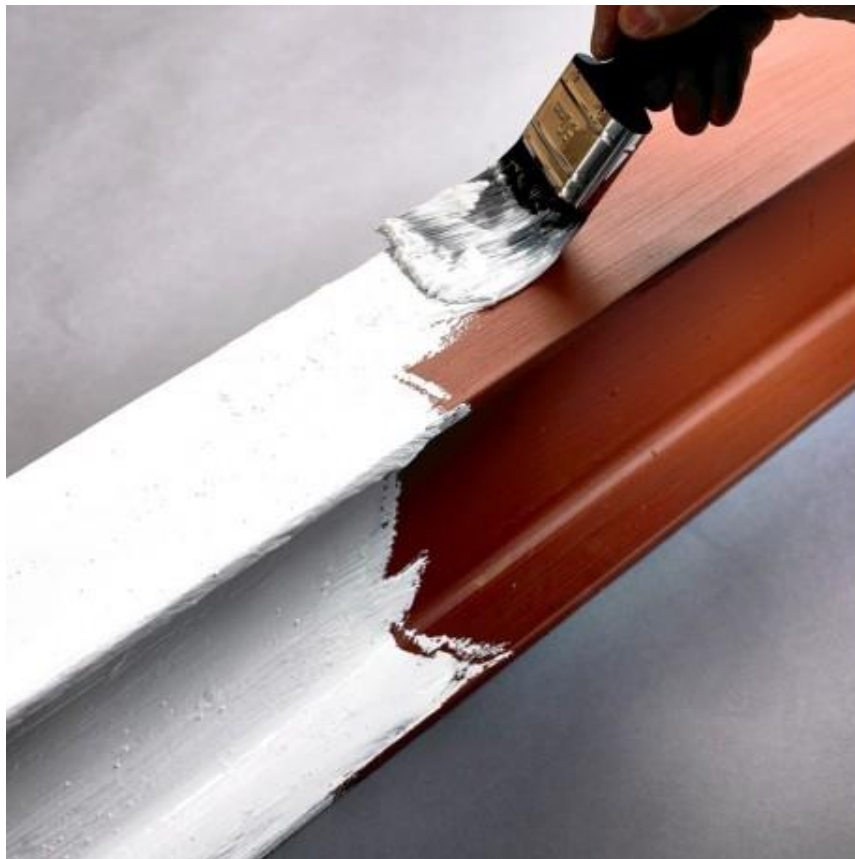
Figure 25 - Covering a steel element in intumescent coating
