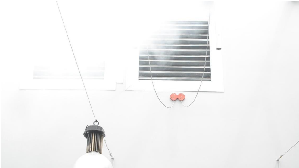
Figure 84 - The mechanical fans exhausting the smoke
