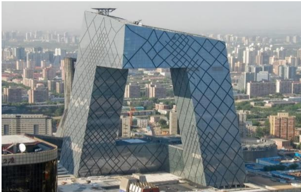
Figure 4 - CCTV building in Beijing, China
