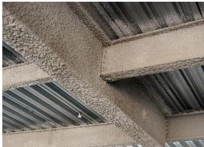
Figure 35 - Steel elements covered in a fire-resistant mixture
