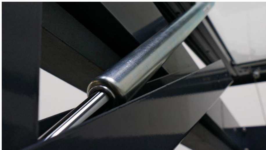
Figure 41 - A servomotor of an automatically opened window
