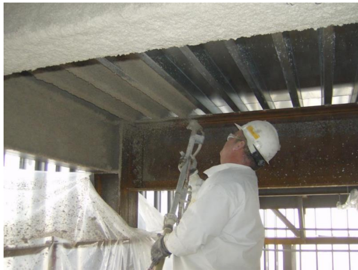
Figure 34 - A worker applying a special fire-resistant mixture on steel elements
