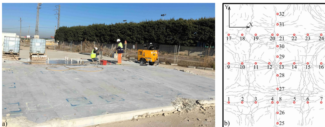
Fig. 14. a) Extraction of cores; b) Numeration of extracted specimens
