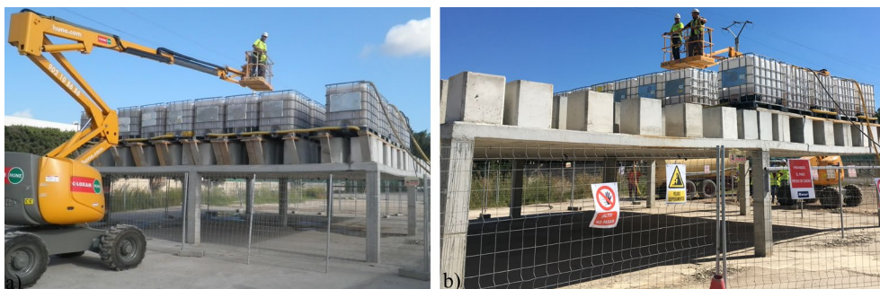
Fig. 9. SFRC slab under ultimate loading conditions: a) loading of the first half of the slab; b) loading of the rest of the slab
