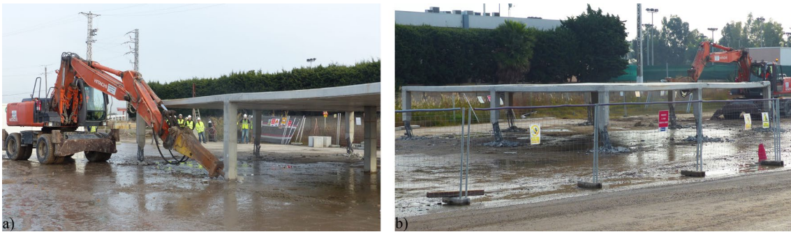
Fig. 8. a) Shattering the column base b) Demolition of the SFRC prototype
