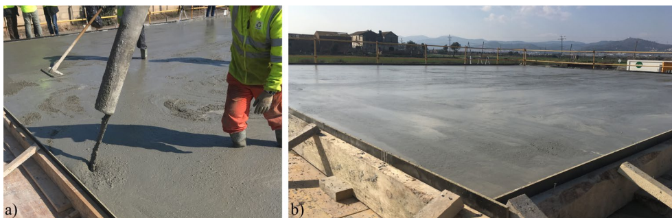
Fig. 7. a) SFRC pumping b) SFRC flat slab in the fresh state
