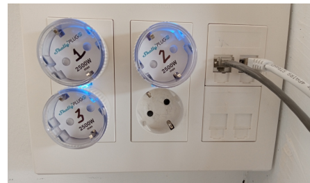
(b) Shelly Plug S installed at Ontec
