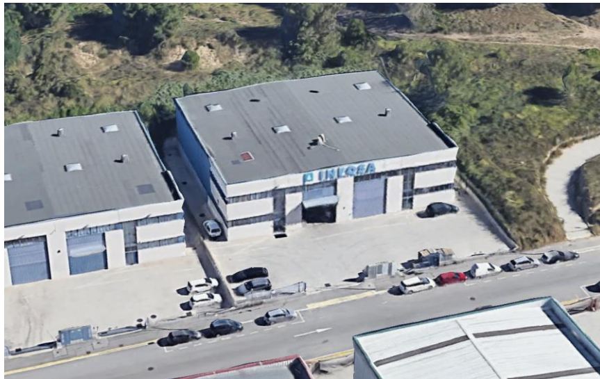
Figure 17 3D view of the building used for the execution of a flat and an unshaded rooftop. [18]
