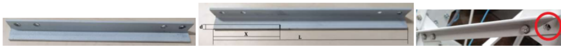
Figure 3. Different structural states of the studied bar. Healthy bar ( left ), cracked bar, where L is the length of the bar, d = 5 mm is the cracked size, and X = L/3 is the location of the crack in the bar ( center ), and unlocked bolt bar ( right ).
