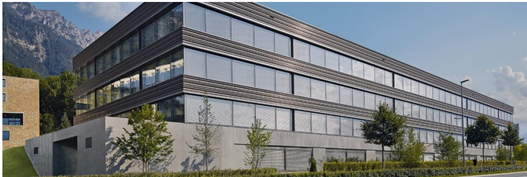
Figure 5.3.1: Picture of the North Office Building located in Hilti HQ in Schaan [62]
