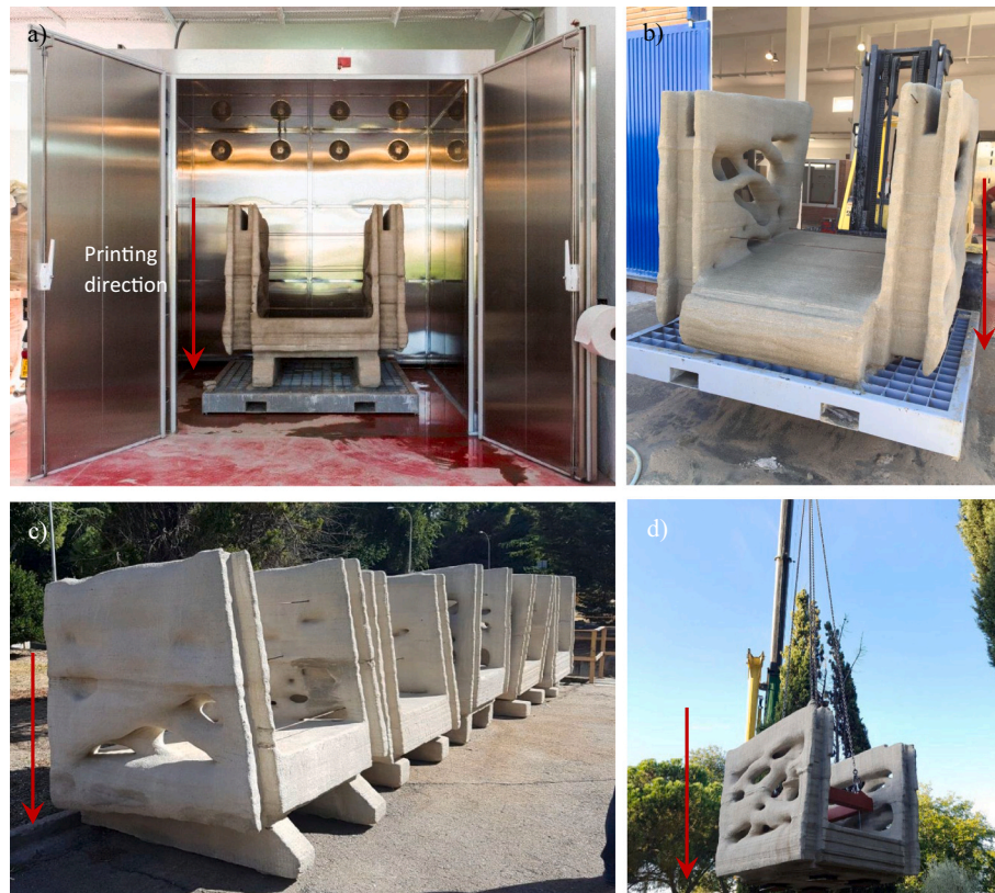
Fig. 18. a) Curing in the temperature-controlled chamber, b) transport of a segment to the external yard, c) curing at external yard environmental conditions, and d) 4-point lifting of the segments with a crane (a red arrow indicates printing direction). (For interpretation of the references to colour in this figure legend, the reader is referred to the web version of this article.)
