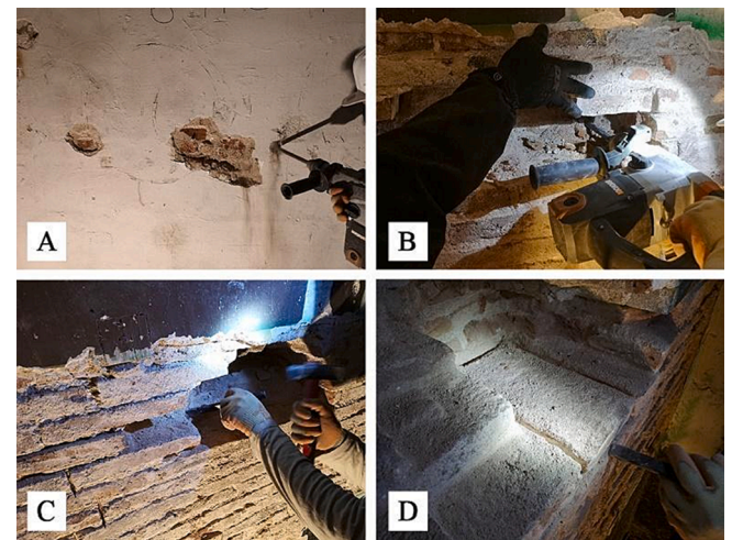
Fig. 3. The extraction process of bricks from existing masonry walls: (A) first, the plaster was removed using a jackhammer; (B) then, the jackhammer was used to break and remove a neighbouring brick; (C) next, a thin chisel was used to remove all the lime mortar joints around the brick; (D) finally, a chisel was inserted under the bed of the brick to lever the brick.
