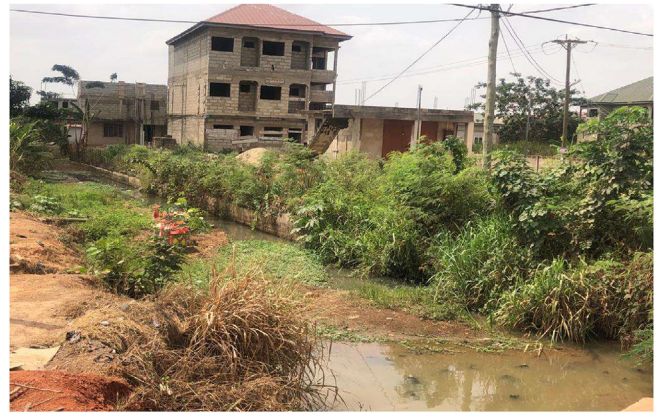
Plate 4. Building on a water course.
