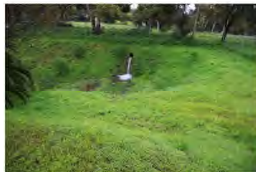
The WGV sump prior to redevelopment, showing typical arrangement, including fencing, weeds, and stormwater flow during a rain event. Source: JBA
