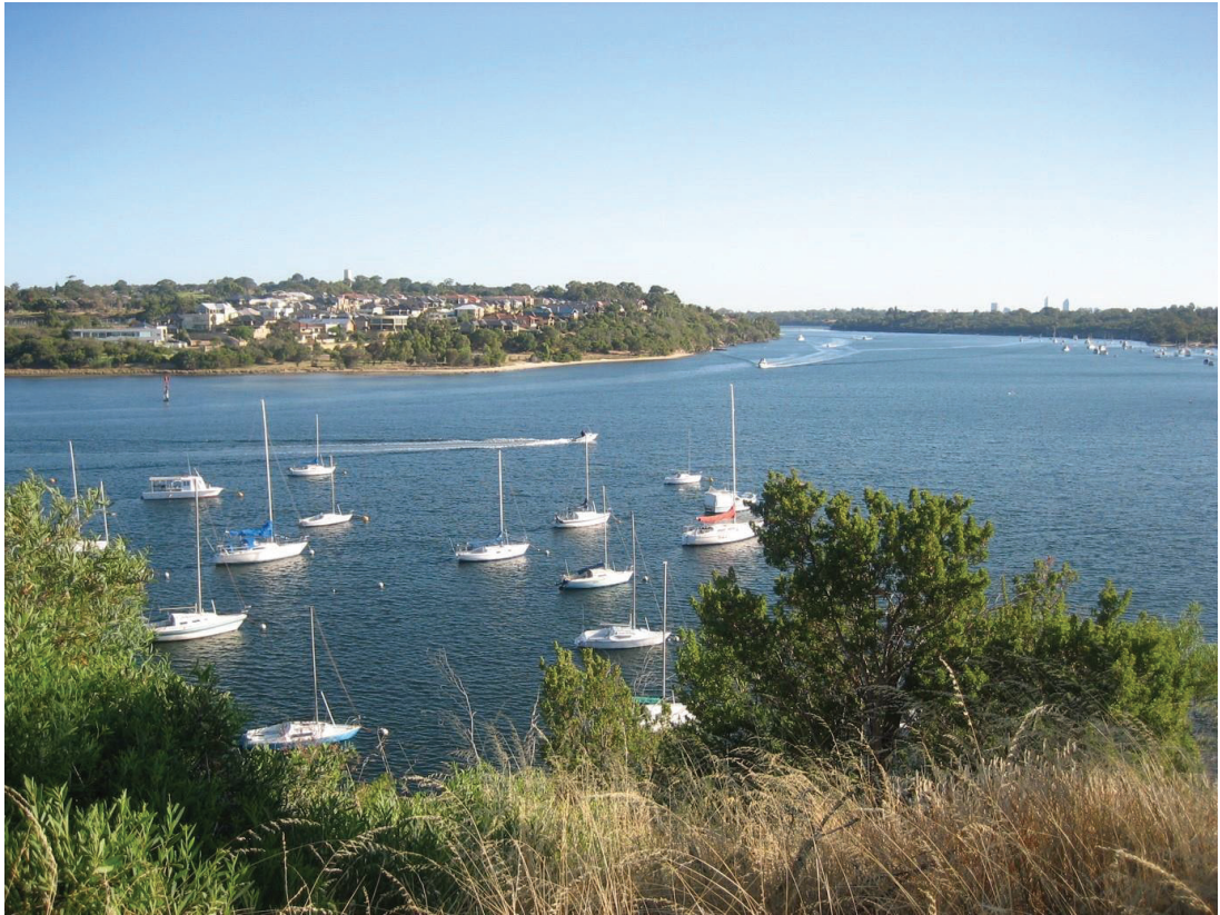
Figure 4. The embankments of Swan River. Credit: Credit: Peter Newman
