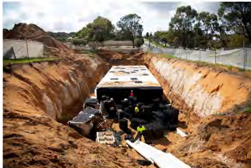
Figure 2. Drainage cells being installed at WGV to ensure adequate drainage function are maintained prior to landscaping. Credit: DevelopmentWA.
