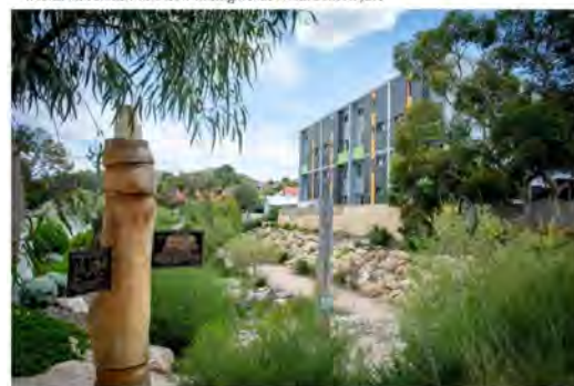
The WGV sump park after completion, with successfully established native vegetation. Source: Rob Frith
