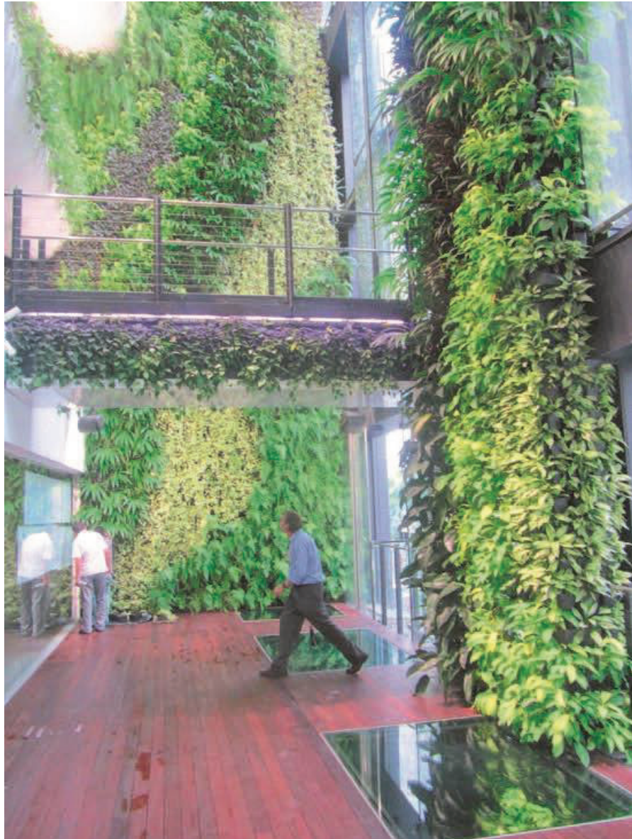
Fig. 5 High-rise green façade in Singapore high-rise office building. Source Photo Peter Newman
