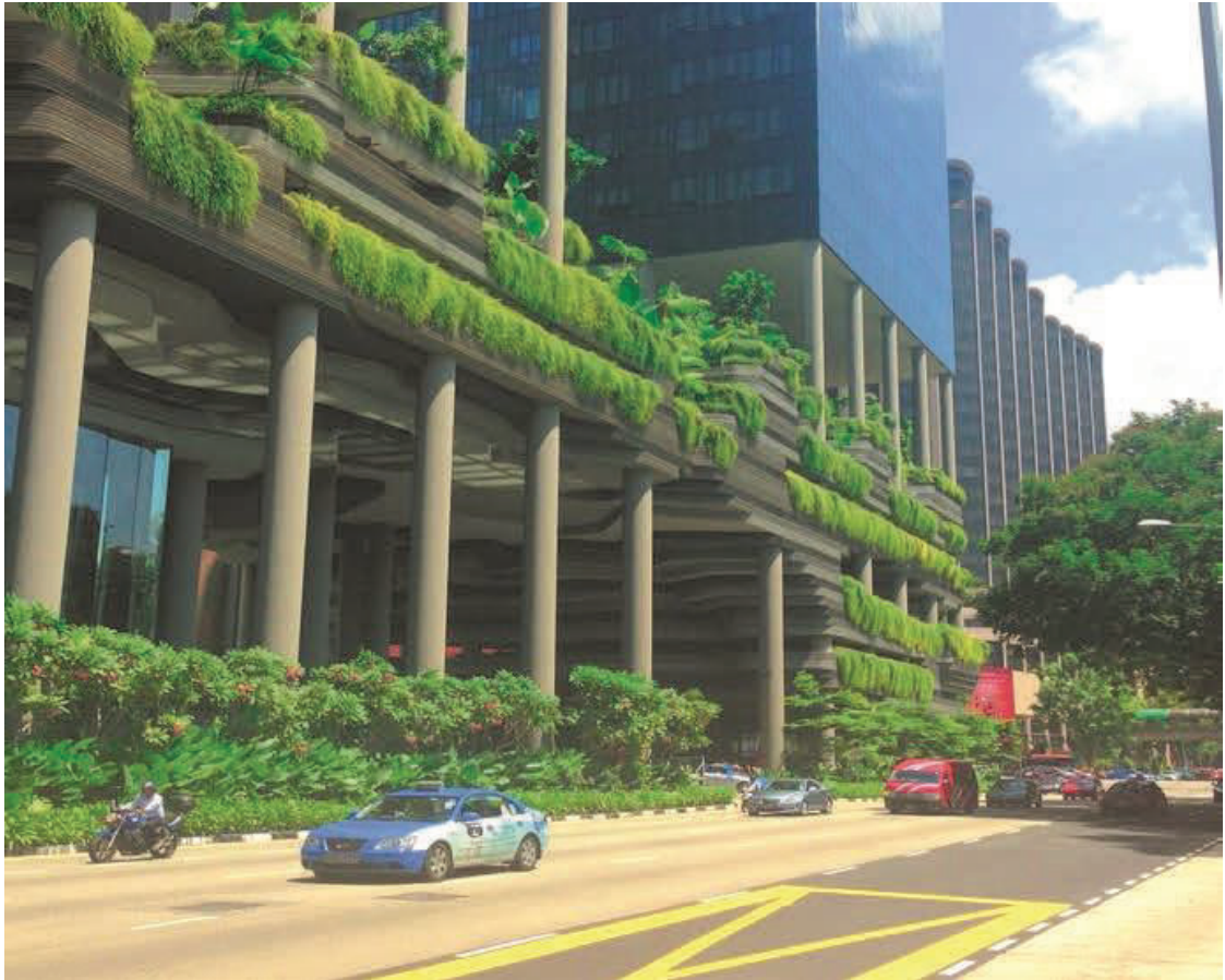
Fig. 2 Singapore's Park Royal Hotel which achieved a green floor ratio of 5:1. (Source Photo
