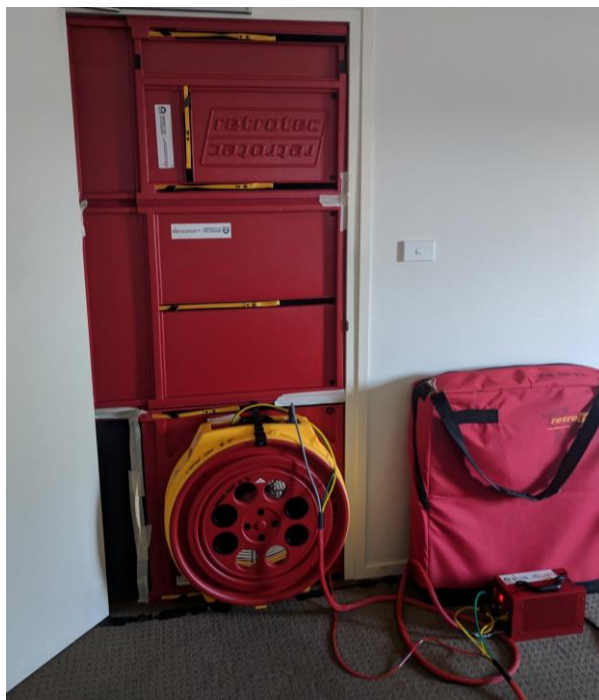
Figure 3-8 Typical blower door setup.
