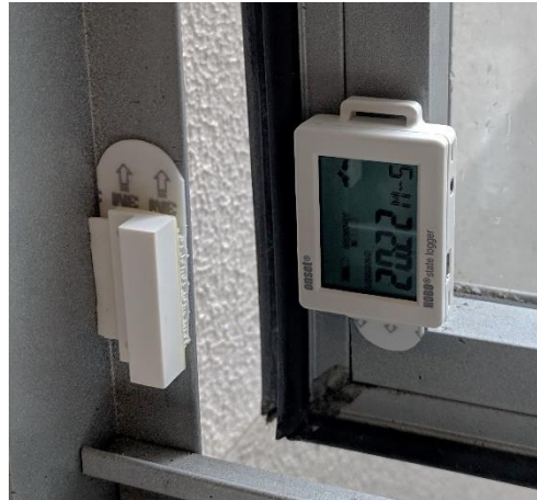
Figure 3-7 HOBO state logger installed on an awning window in opened position
