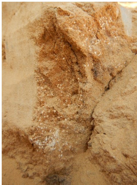
Figure 6.11. Photograph of OSL Cut 1L and detail of salt mineralisation (white specks) and termite frass (dark sediment) at the base of the section's eastern wall, close to the surface.
