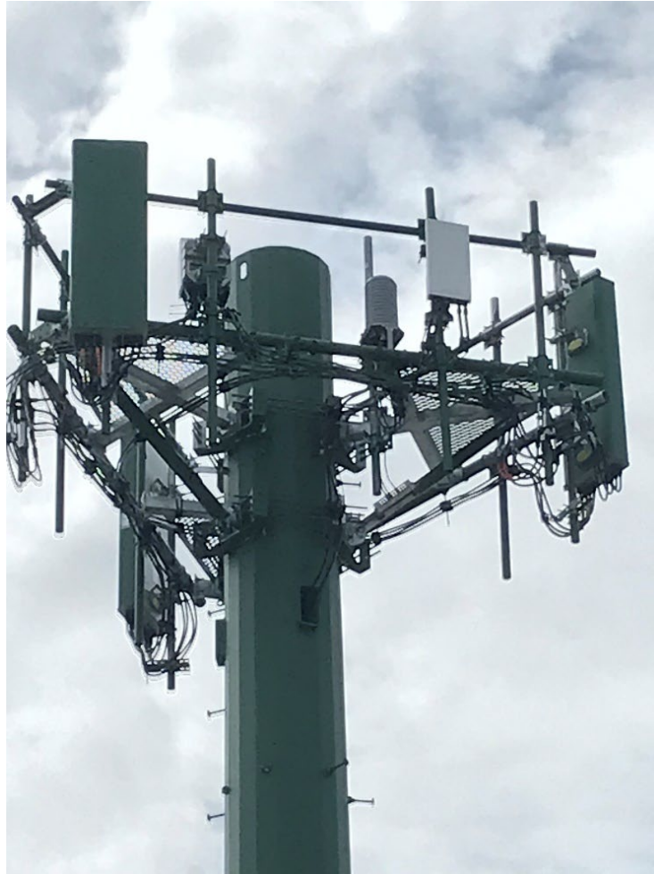
Figure 6. AT&T 5G 50-ft Millimeter Wave Tower. Source: LCDR Caplan iPhone (2022).
