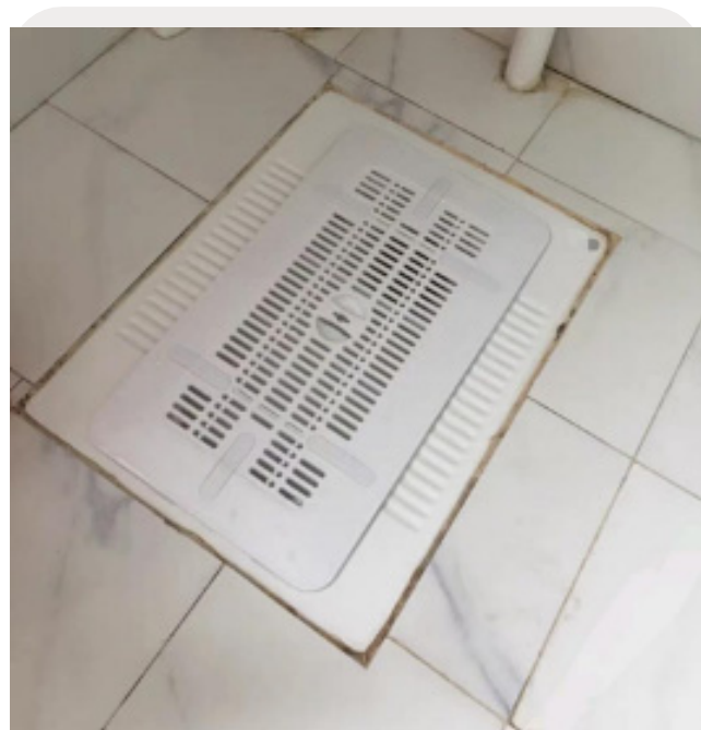
Fig. 1. A multigrad hand-controlled toilet cover to prevent objects from dropping into the toilet when not in use.
