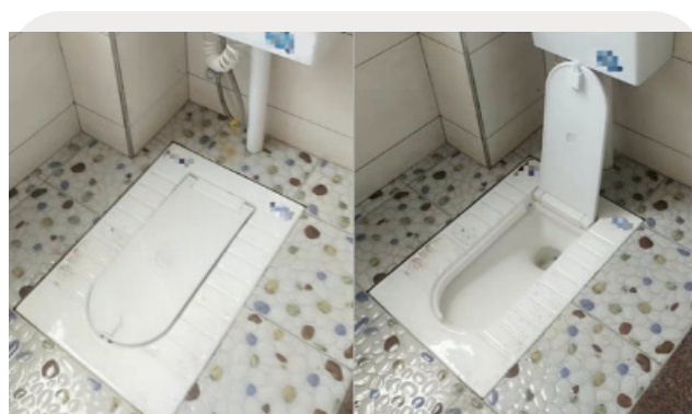
Fig. 2. Domestic squatting toilet with a foot-controlled cover.
