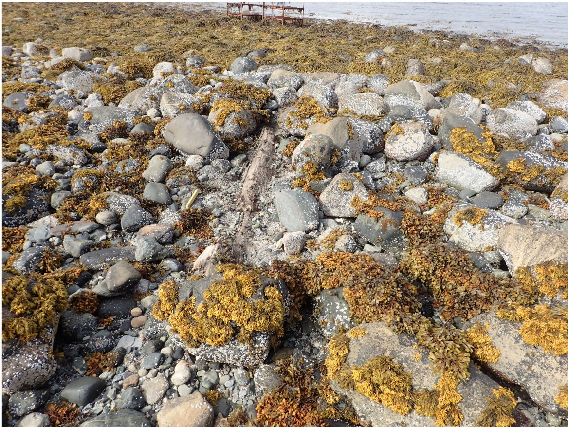
Figure 6. North facing picture showing the location of part of the King Øystein’s harbour’s structure in the intertidal zone which poses challenges of protection and management. The log in the centre of the image is 1.25 m in length and it was originally a part of the base of one of the wooden caissons that constituted the breakwater. Photo: Fredrik Skoglund, NTNU University Museum.
