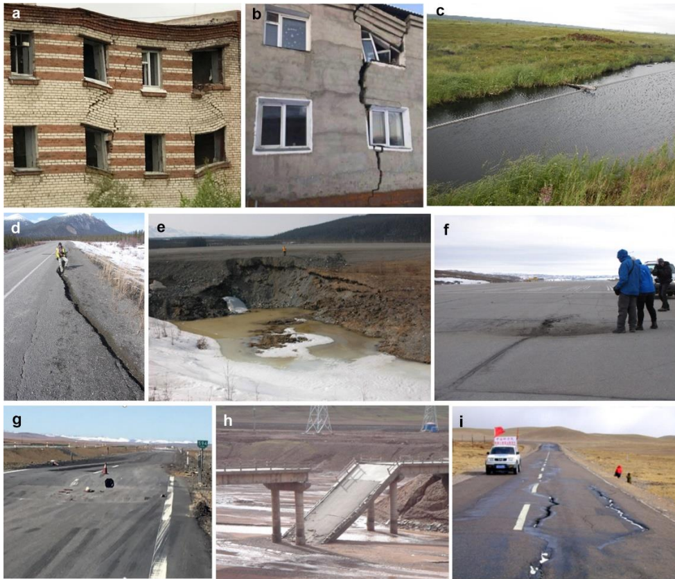
Fig. 3. Infrastructure damages owing to degradation of permafrost. a and b Damaged buildings due to permafrost degradation in Yakutia, Russia (Photos by Ivan Khristoforov). c Below-ground pipeline in crossing an area with ice-rich permafrost and thermokarst development in Yamal-Nenets, Russia. d Longitudinal cracking due to shoulder rotation along the Alaska Highway in Yukon, Canada. e Thermokarst affecting partly the embankment of the Alaska Highway in the Yukon, Canada (Photo by Eva Stephani). f Sinkhole in the Iqaluit runway (Nunavut, Canada). g Embankment deformation of the Gongyu express highway, China (Photo by Chen Ji). h Collapsed bridge of Qinghai-Tibet Highway, China. i Longitudinal cracks of Qinghai-Tibet Highway, China.
