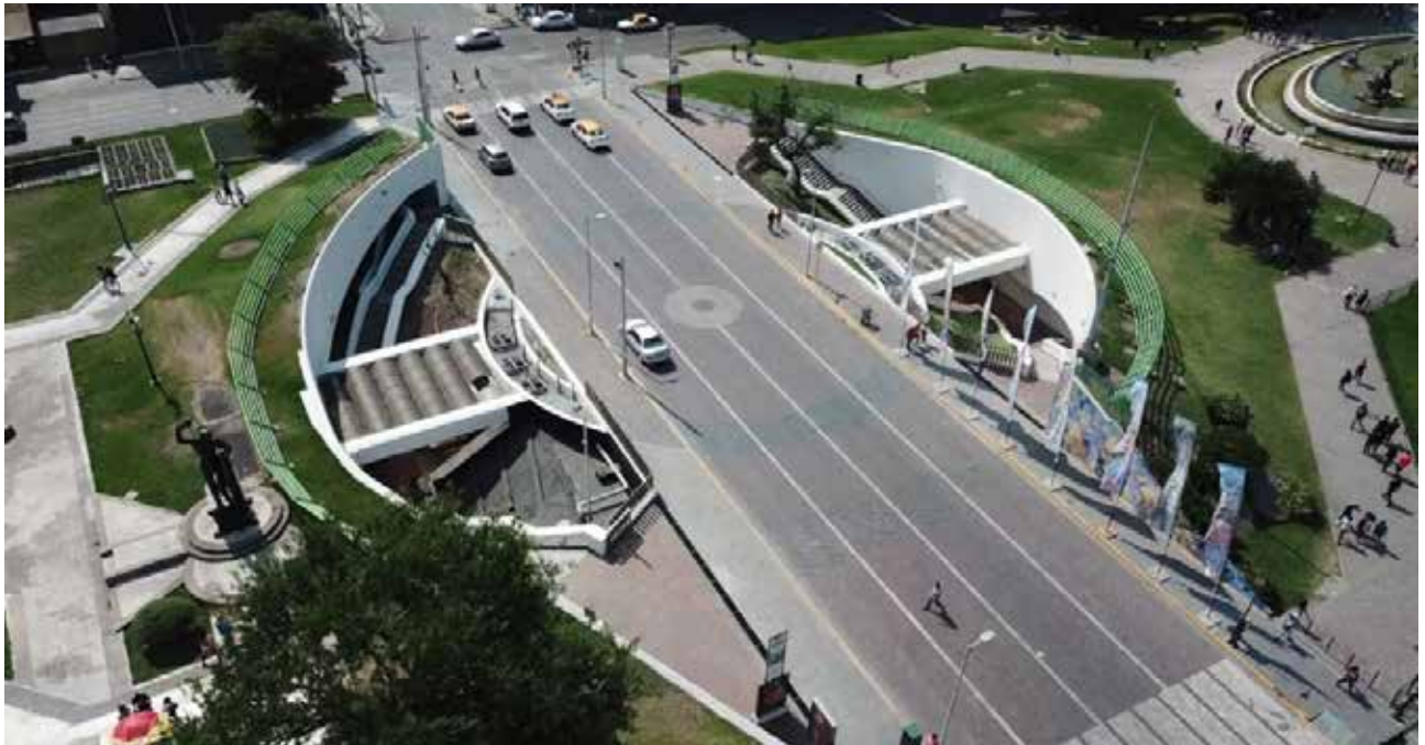
Figure 20. Aerial view of the entrance of Zaragoza station, photo taken by The Raws (2021)
