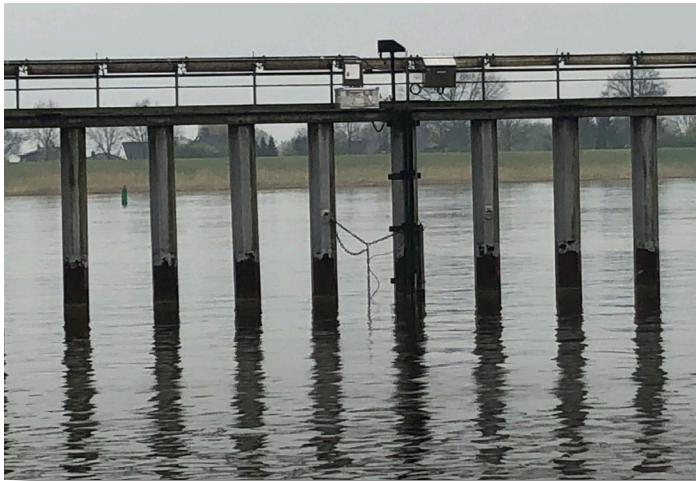
Fig. 5.4: Deployment of the methane sensor in Geesthacht, AKW pier; the Zarges box with computer and WLAN router can be seen at the “bridge” with chains and the sensor attached going downward. (Photo: A. Krönert)
