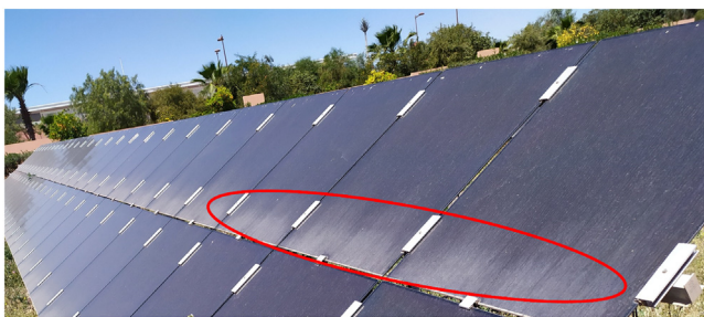
Fig. 5. Soiling distribution on a PV system installed at the Green Energy Park.
