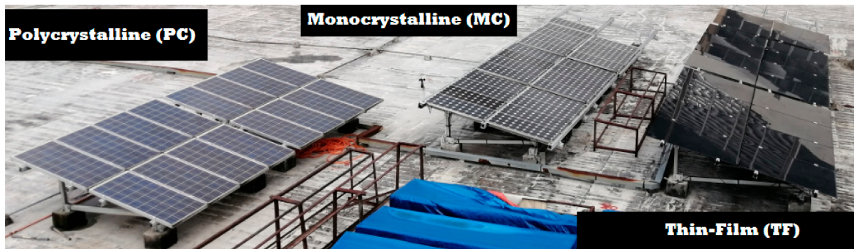
Figure 4. Three PV systems on the engineering tower's roof at the University of Malaya.
