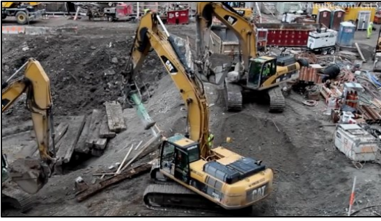
(a) Two backhoes loading trucks and hammering
