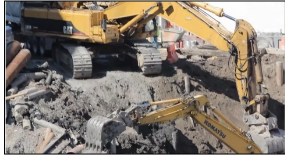
(b) Two backhoes working in a tight area
