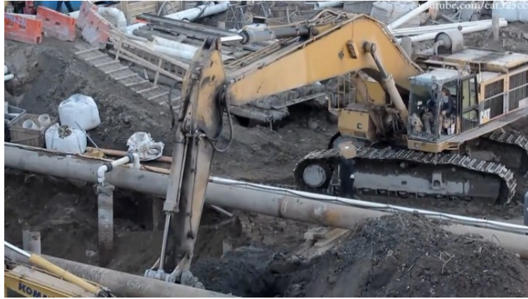
Figure 4.1 Excavator digging between two pipes in a congested site
