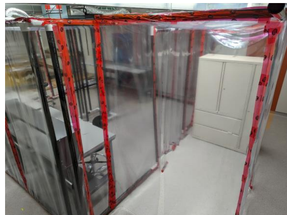
Figure 3: An Intermediate Space Between the Unfiltered Laboratory Space and the Cleanroom Door
